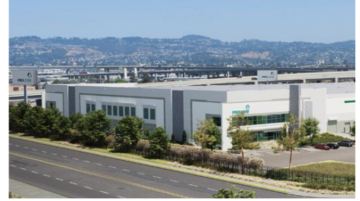
Phase II - State of the Art Class "A" Warehouse Development Under Construction
