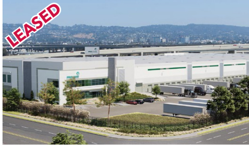
Phase I - State of the Art Class "A" Warehouse Development
