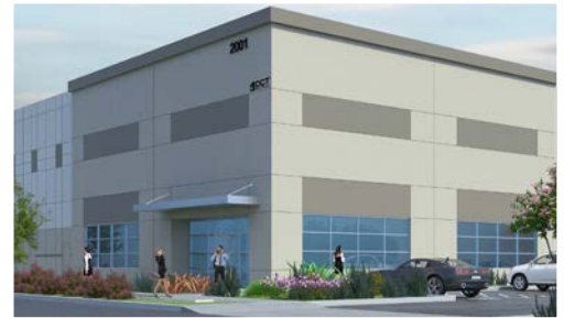
Under Construction Class "A" Warehouse
