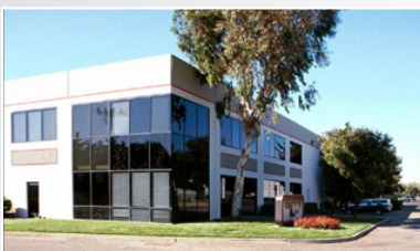
Industrial - 69,438± SF Leased 3875 Bay Center Place, Hayward ALAMEDA ELECTRIC
